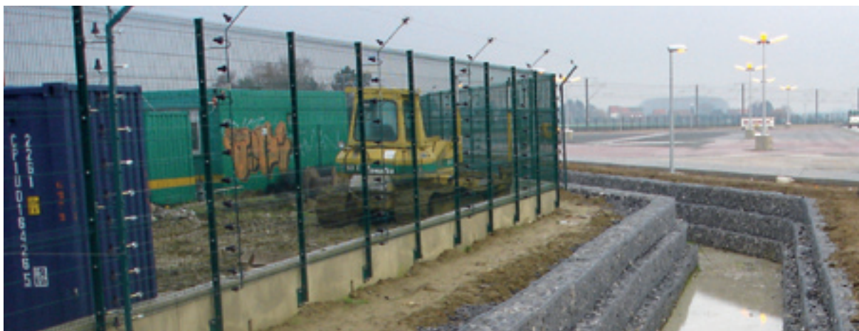
Parking D'Ieteren – Belgia – Securifor® + Gabiony
